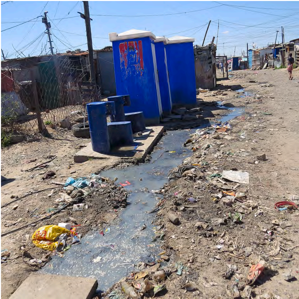
Fig. 5. John's photograph, "Leaking tap".
